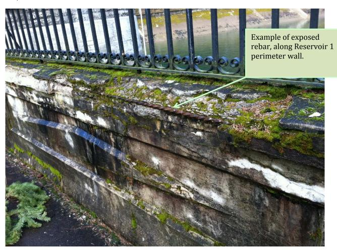
Much of the raised decorative diamond pattern has been lost. The wall cap has been lost in places and more is lost every day. The concrete sits in chunks on the ground. Much of this south wall will need to be reconstructed.
