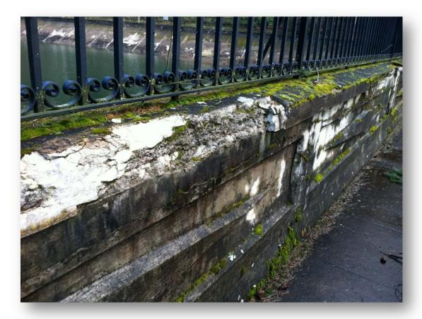
Other examples of neglect include the lack of periodic cleaning to remove damaging mold on the reservoir walls and neglect in patching holes in the masonry.
